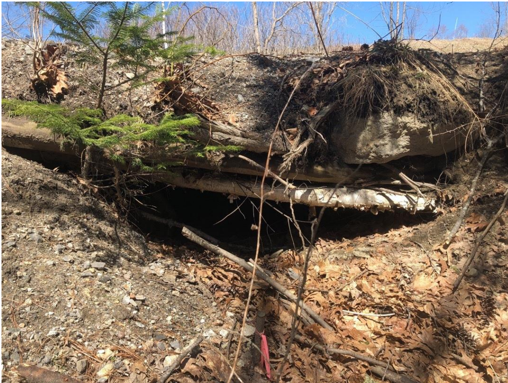
Photo 8. South of Olive Avenue Medium severity erosion beneath rail.
