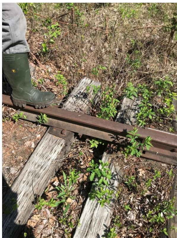
Photo 15. Near Old Lisbon Road Minor erosion beneath rail.
