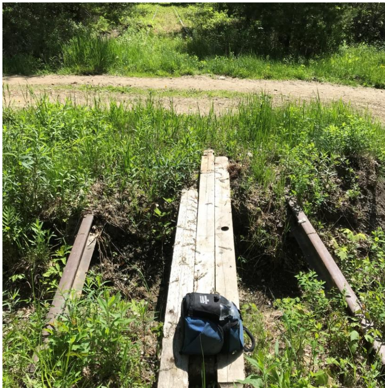
Photo 16. Between Old Lisbon and Crowley Roads Medium severity erosion beneath rail.
