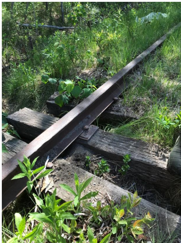
Photo 12. East of Turnpike Overpass Minor erosion beneath rail.
