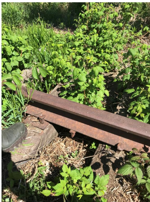
Photo 13. East of Gould Road Minor erosion beneath rail.
