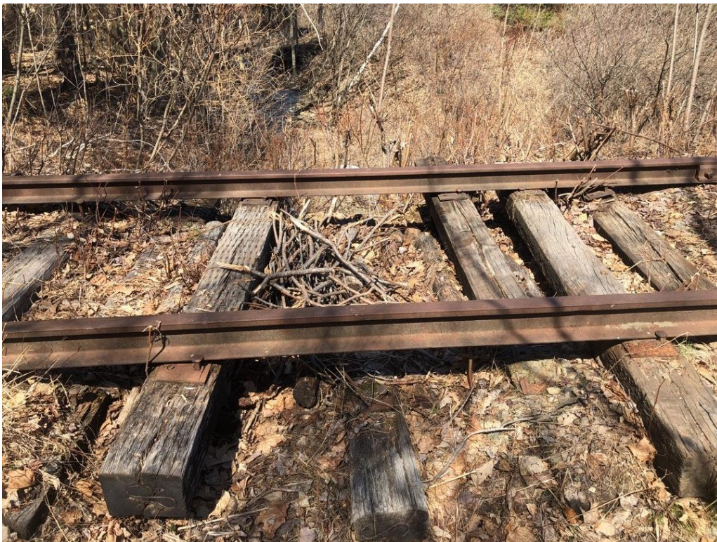
Photo 9. West of Liberty Mutual Medium severity erosion beneath rail. Wetland and stream in background.
