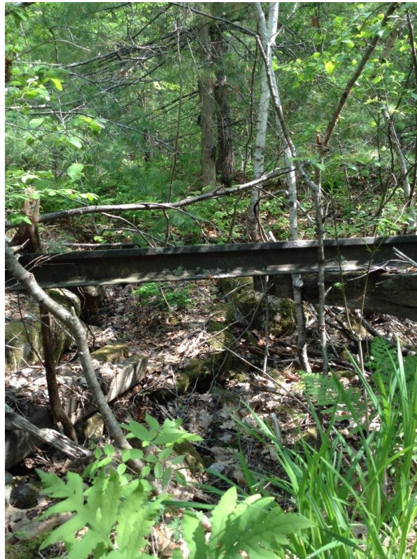
Photo 18. West of River Road, Lisbon Severe erosion beneath rail.
