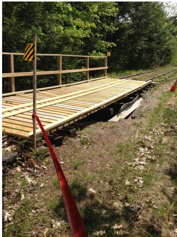
Photo 19. Near River Road, Lisbon Severe erosion beneath rail resulted in a pedestrian bridge.
