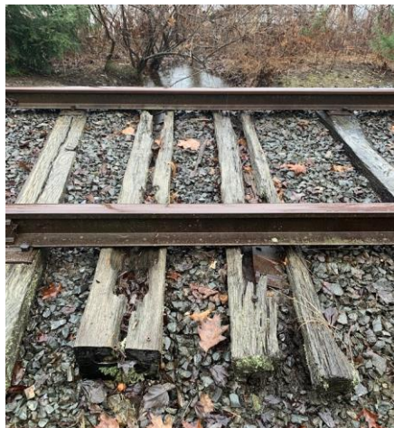
Figure 4: Typical failing crosstie
