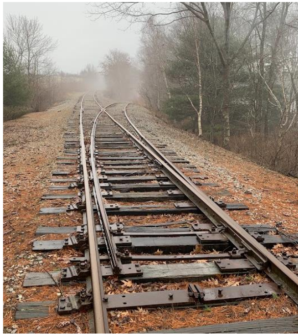
Figure 7: Turnout to Grimm Industries Siding
