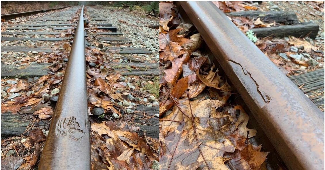
Figure 6: Typical Rail Wear
