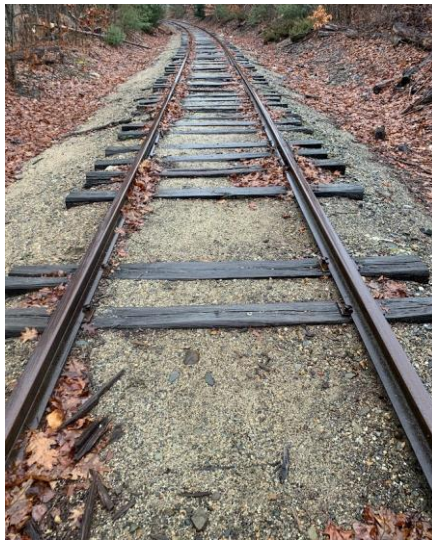
Figure 5: Gaps in cross tie spacing
