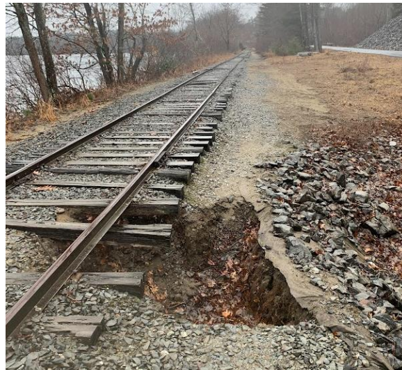
Figure 2: Typical Washout
