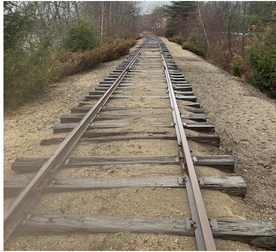
Figure 3: Fouled Ballast (Lisbon)
