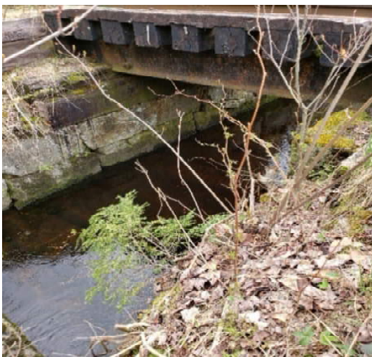
Figure 8: Red Brook Bridge – Stone Abutment with Timber Seat and Steel Stringers Arch Culvert Barrel
