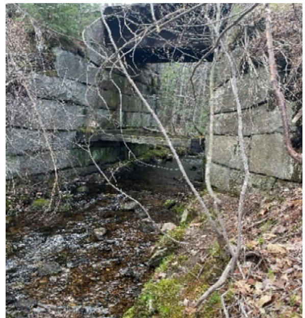
Figure 15: Pierce's Brook Bridge – Stone Abutment with Timber Strut Supports
