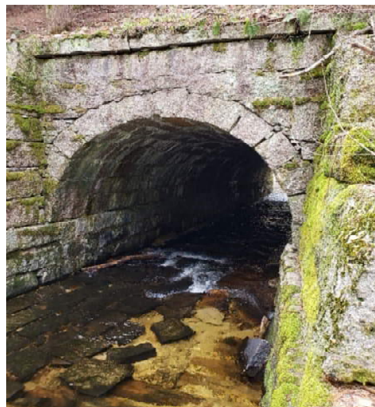
Figure 11: Break Neck Brook Bridge – Stone Arch Culvert Headwall
