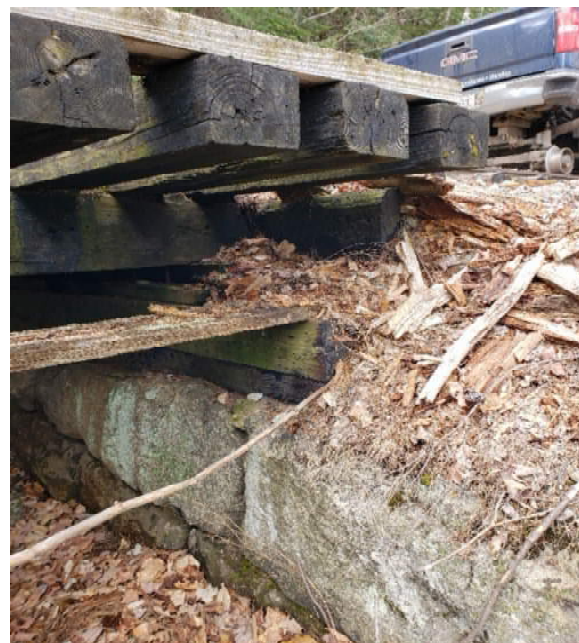
Figure 13: Cattle Pass Bridge – Stone Abutment with Timber Stringers and Ties
