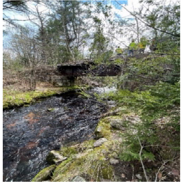
Figure 18: Little Saco River Bridge – Stone Masonry Abutment and Steel Girder Superstructure
