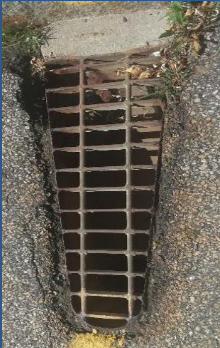
Drain Gate (Erosion Present)
