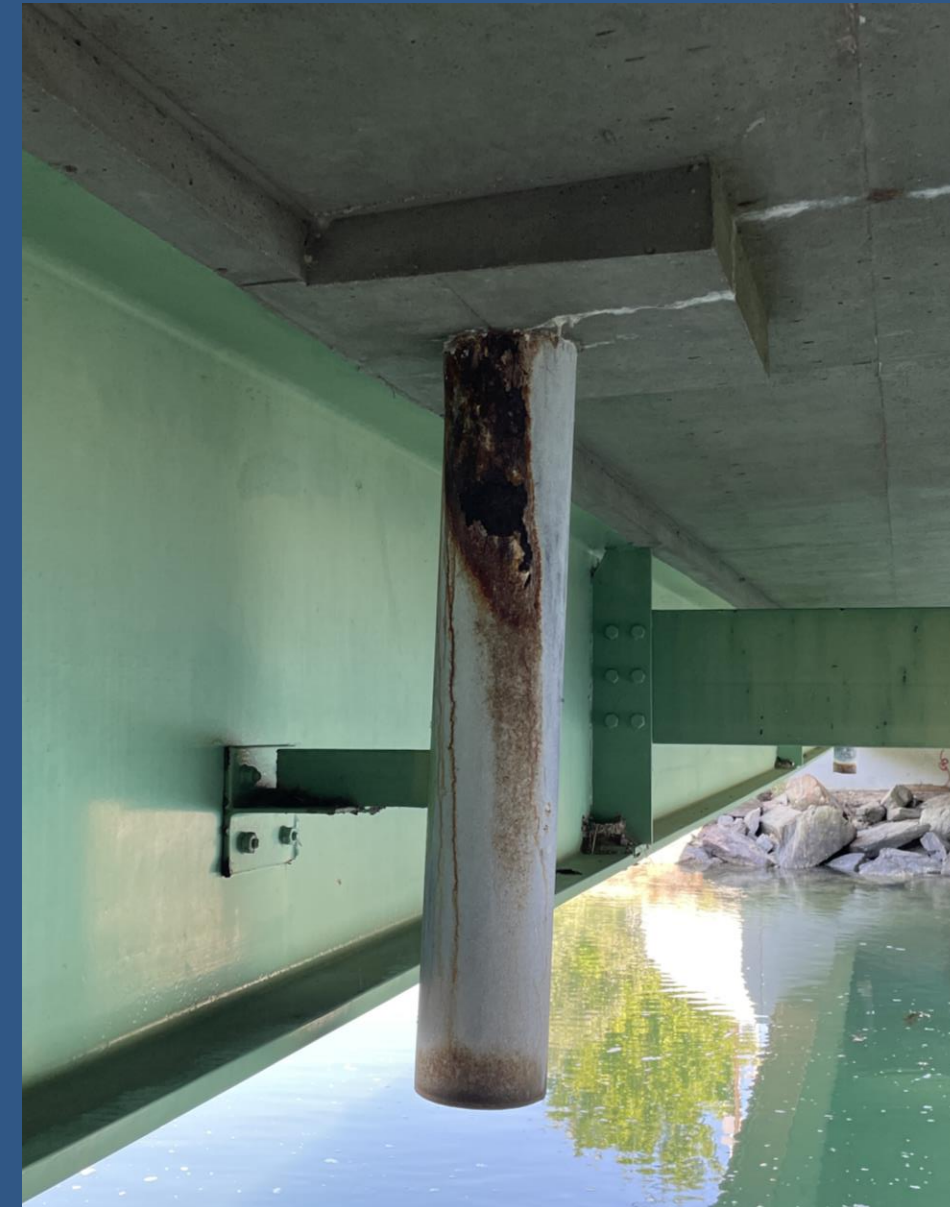
Drain Downspout (Rust Present)
